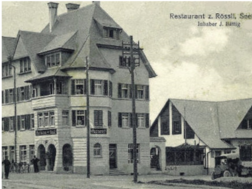
Rest. Rössli, Zürich-Seebach (1913)
